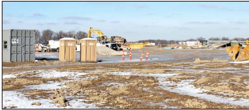
Construction on Crown Lift Trucks' new facility in Maumee
